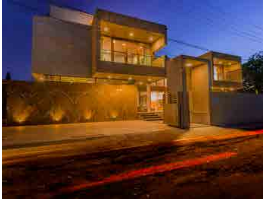
Intuitive night time illumination takes front stage in the definition of the elevation features, helping the residence stand out and have a strong identity.
